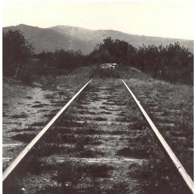
End of the rail line in Victor, Idaho
