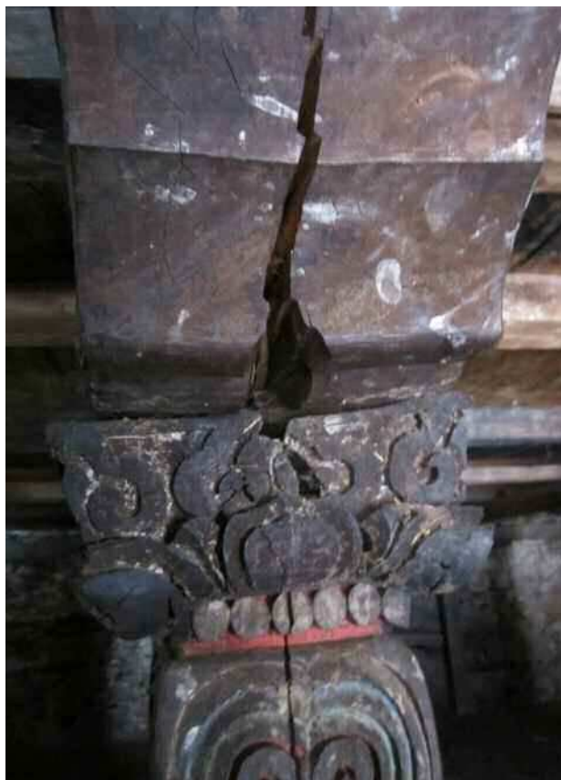
Figure 4. The weight of the roof is causing the carved wooden interior supports to crack.
