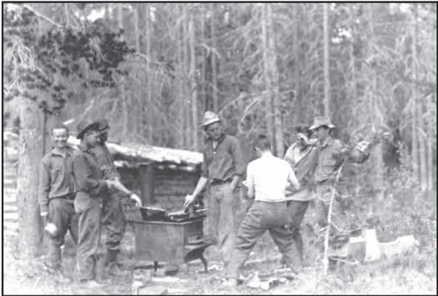
Jackson Lake Dam crew cooking supper, c. 1915 1958.0773.001
