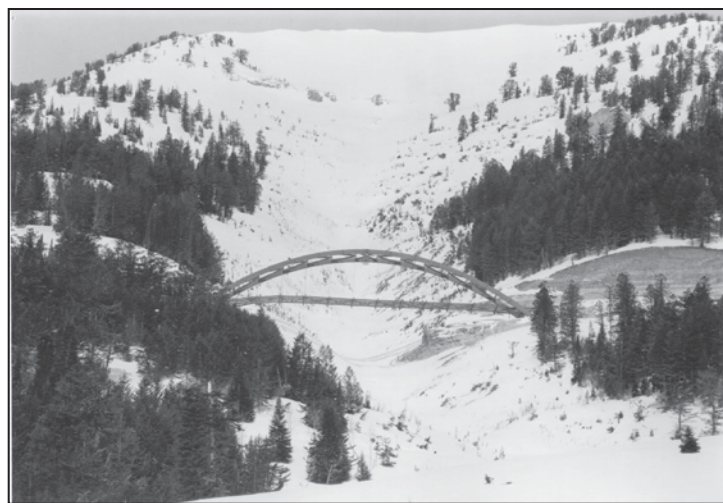
Crater Lake Bridge Courtesy of Wyoming Department of Transportation
